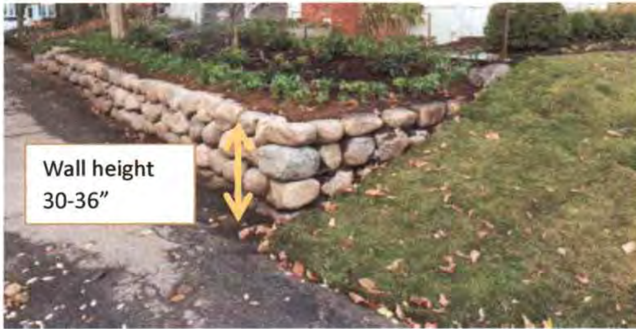
Figure 7 Proposed front retaining wall to match image above. The wall will be 30 -36 inches tall.
