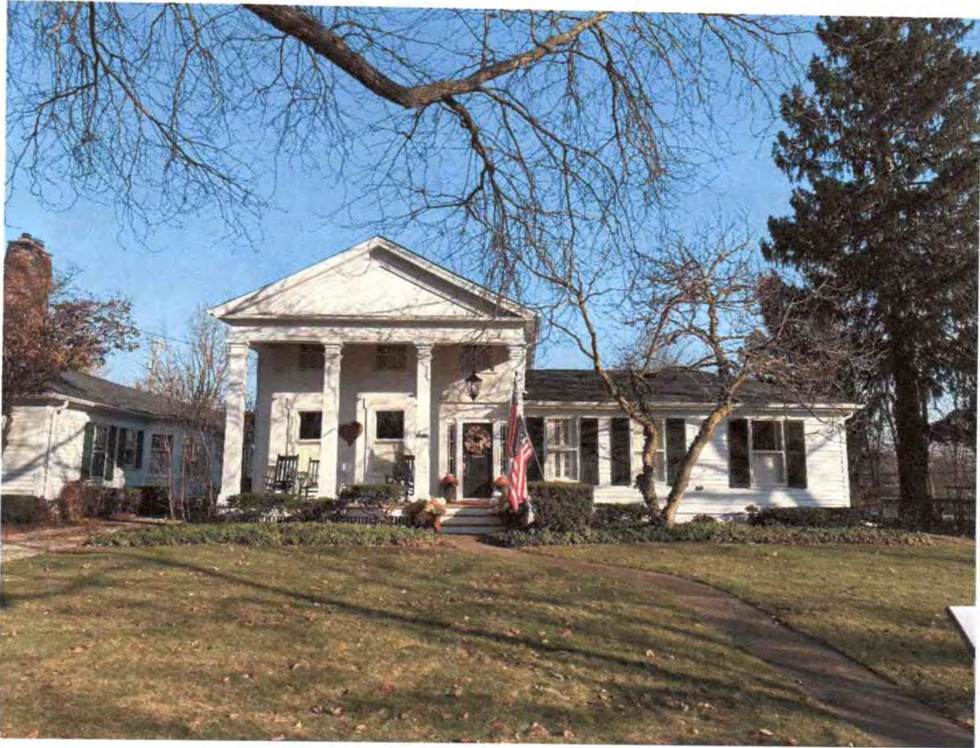
Figure 1 Front elevation of existing home
